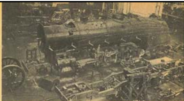
Cylinder saddle attached, boiler, firebox is lowered on frame.
