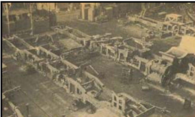
Basic cast frame bed for future 141R 121 on erecting floor.
